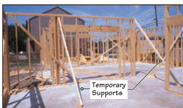
FIGURE 5 Wall assembly under construction.
