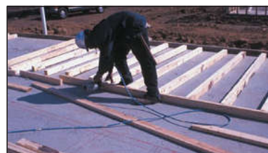
FIGURE 6 Walls are typically framed on the slab or floor platform and subsequently tilted up into position.
